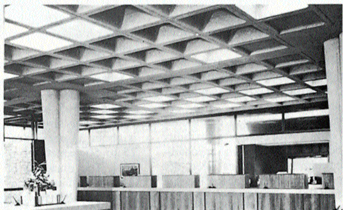
Waffle plate two-way structural system
