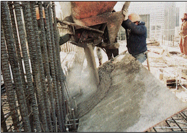
Superplasticized concrete dumped from bucket against plywood panel flows into forms where heavy reinforcement has been set. Extended-life superplasticizer helped speed crane-and-bucket placement at the 58-story Trump Tower on Fifth Avenue.
