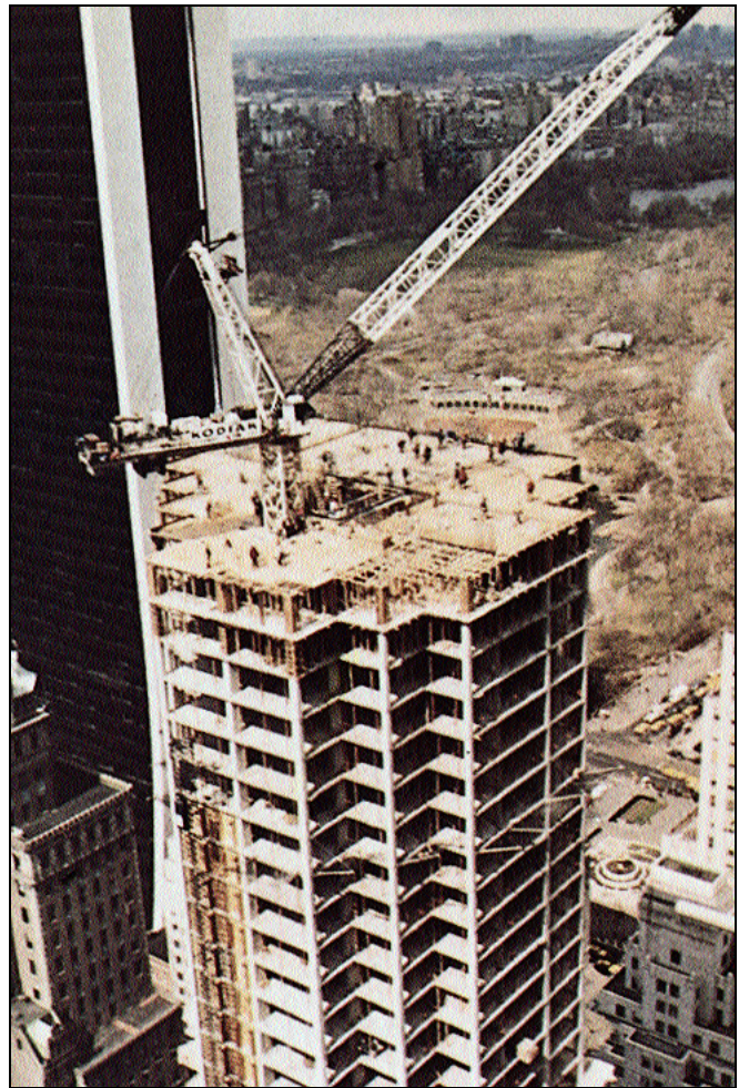
Tower crane located off center at Trump Tower lifted forms and reinforcement, then with bucket attached placed concrete on a two-day cycle for the 11,700-square-foot residential floors.
