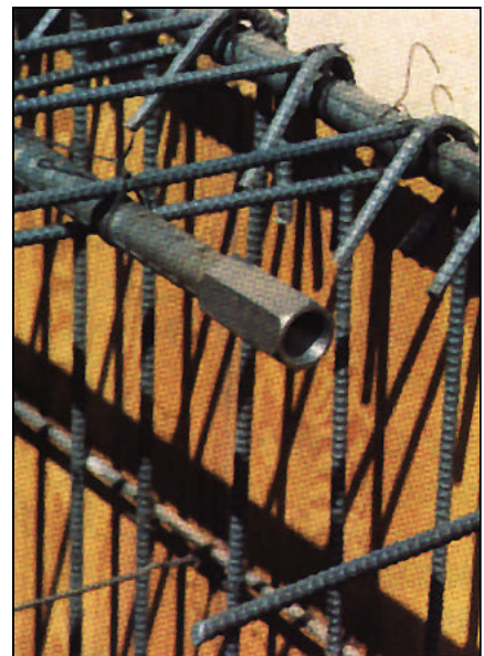
Figure 4. This system's taper-threaded coupler is used to butt splice two lengths of rebar, each threaded to match the coupler. The mating bars (not shown here) will be placed in the couplers, rotated by hand, and tightened with a pipe wrench.
