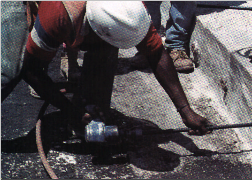
Figure 3. To secure a construction-joint connection, workers must insert the mating bar into the exposed end of the coupler. Encased in the concrete is the coupler, as well as the bar that was previously attached to the coupler.
