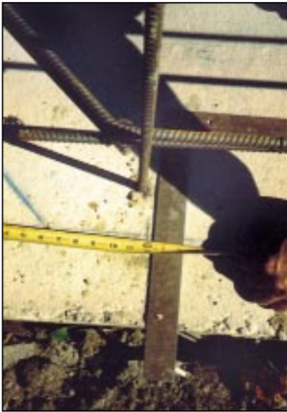
Figure 3. To determine the size of filler needed, measure along the chalk line from the carpenter's square to the edge of the hinged corner.
