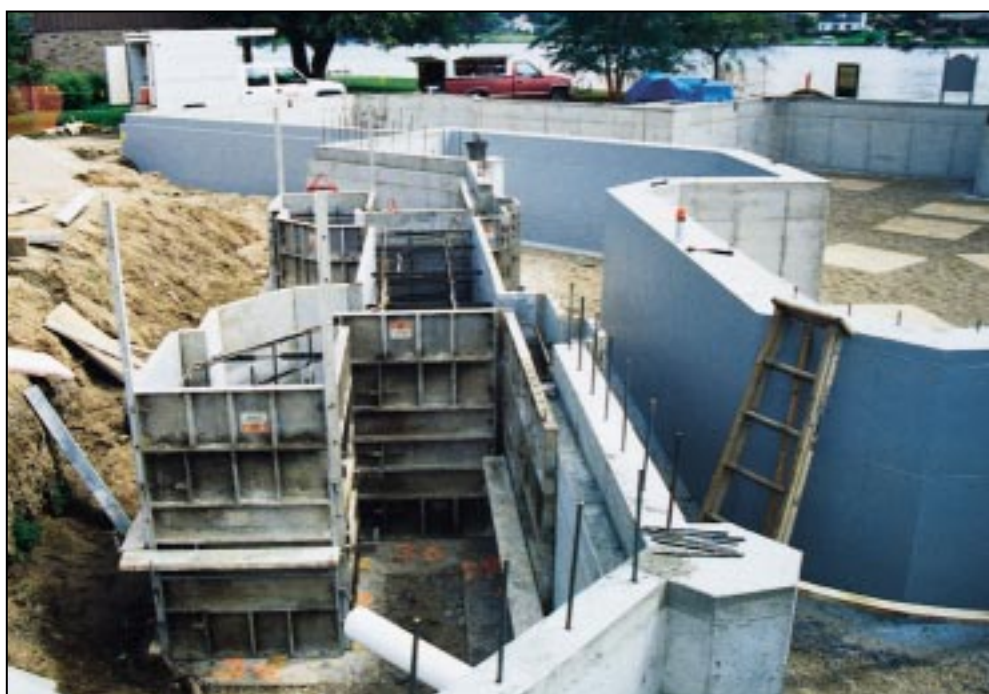
Multiple wall thicknesses and corner angles, uneven dimensions, and a brick ledge were some of the complexities and challenges of building this residential basement.
