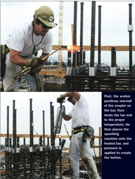
of the bars to be spliced. The hydraulic pump (which the user provides) must be rated for 10,000 psi. For heating, a gas mixture of propane and oxygen is recommended, although other mixtures, such as acetylene and oxygen, may be used.
