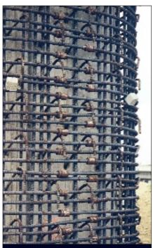
The Xtender is being used in California to create continuous hoop steel for retrofit of the columns on elevated freeways. For hoops, the couplers can be used on rebars up to #8.
