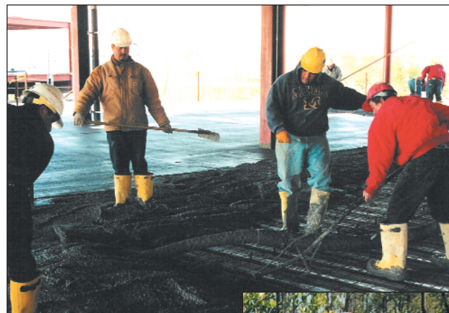
Right: Paul Albanelli of Albanelli Cement Contractors of Farmington Hills, Mich. Albanelli is a family-owned company with over 50 years of concrete construction experience. Above: The crew places lightweight concrete on an elevated slab.
